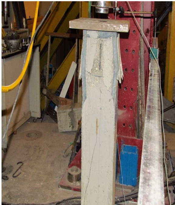
Figure 4-6: Failure of column C21
