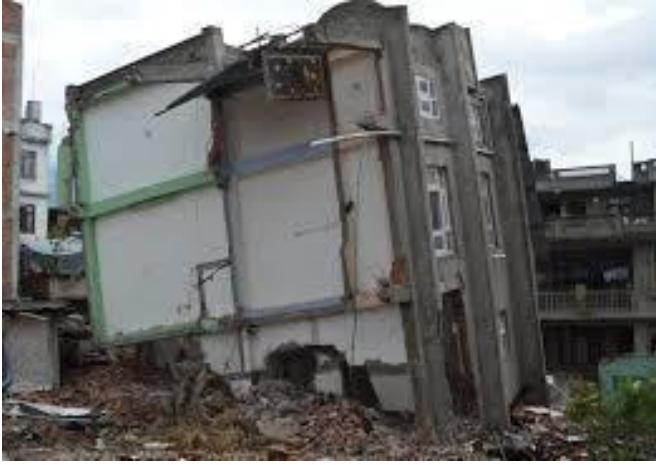
Figure 1-2: Building Collapse due to an earthquake in Nepal ( www.concrete.org )
