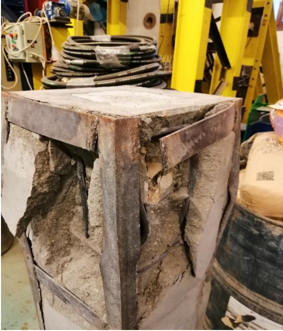
Figure 4-12: Failure of column C51
