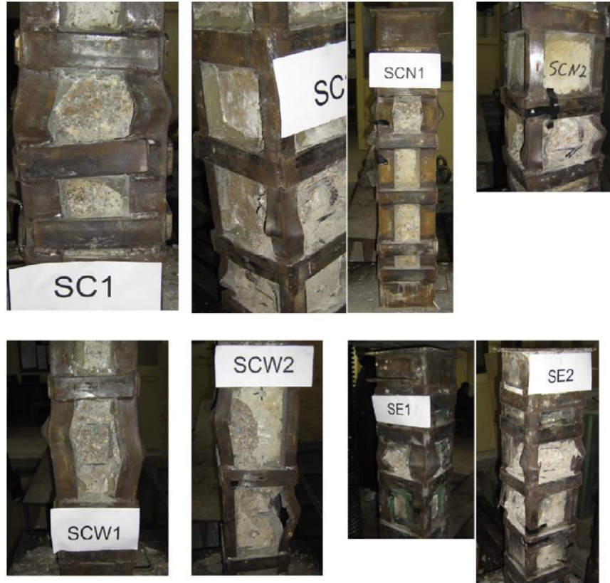
Figure 2-10: Failure Shape of strengthened columns (Tarabia, 2014)
